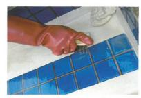
3 – Scrub the surface vigorously using a wire brush and flush with clean water. Leave to dry for at least 3 hours.
