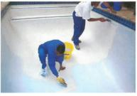
3 – Apply the first coat in one continuous operation to avoid dry joints. Do not stop and start. Do not patch, Leave to dry for at least 3 hours.
