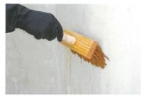
2 – Apply the acid mix to the surface using a blockbrush.
