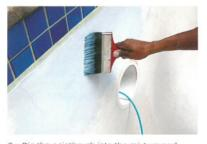
2 – Dip the paintbrush into the mixture and brush the surface liberally. Be sure to fill small holes and indentations.
