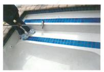
6 – Brush and vacuum surface to remove all dust. Mask where there is a risk of splashing and where straight edges are required.
