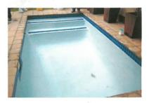
6 – Leave the completed pool to air-cure for 6 days. In case of rain during this period, remove any water from the floor of the pool.
