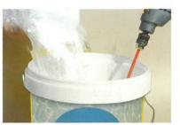
3 – Slowly add the powder from the plastic bag while stirring. The mixture should be smooth with no lumps. A small amount of water may be added if required.
