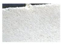
5 – The surface should be very rough to the touch. If this is not the case, repeat the acid washing procedure described above.
