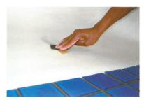
4 – Remove high spots and calcium build-up using 80 grit sandpaper. Be sure to remove any loose materials.
