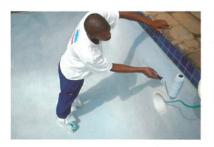
4 – Apply the second coat using a sheepskin roller. Ensure that the first coat is properly covered.
